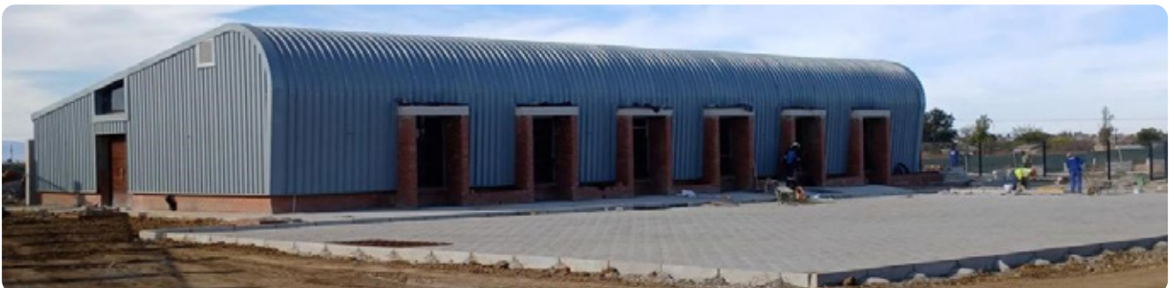
Construction of Clothing and Textile Hub at Madadeni Industrial Estate
