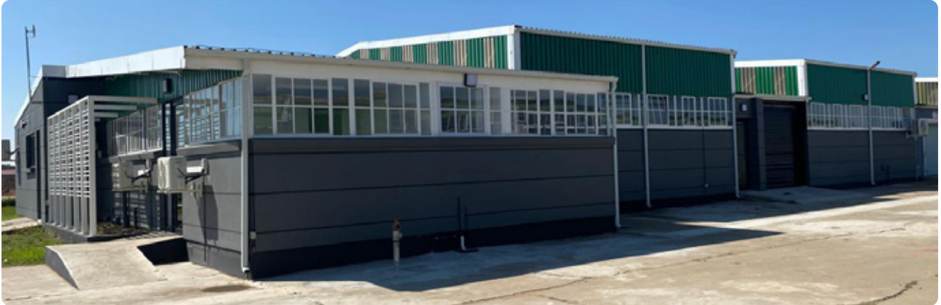
Detergents Shared Manufacturing Facility situated in Amajuba District Municipality
