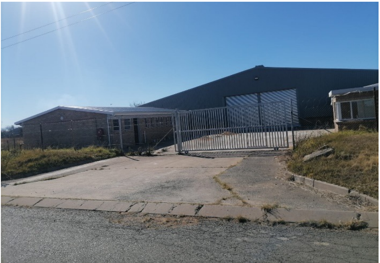
Rebuilt Factory at the Madadeni Industrial Estate
