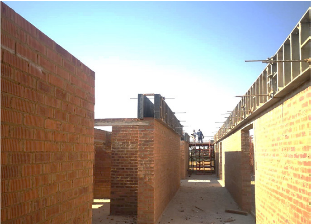
Madadeni Clothing and Textile Hub Construction Progress
