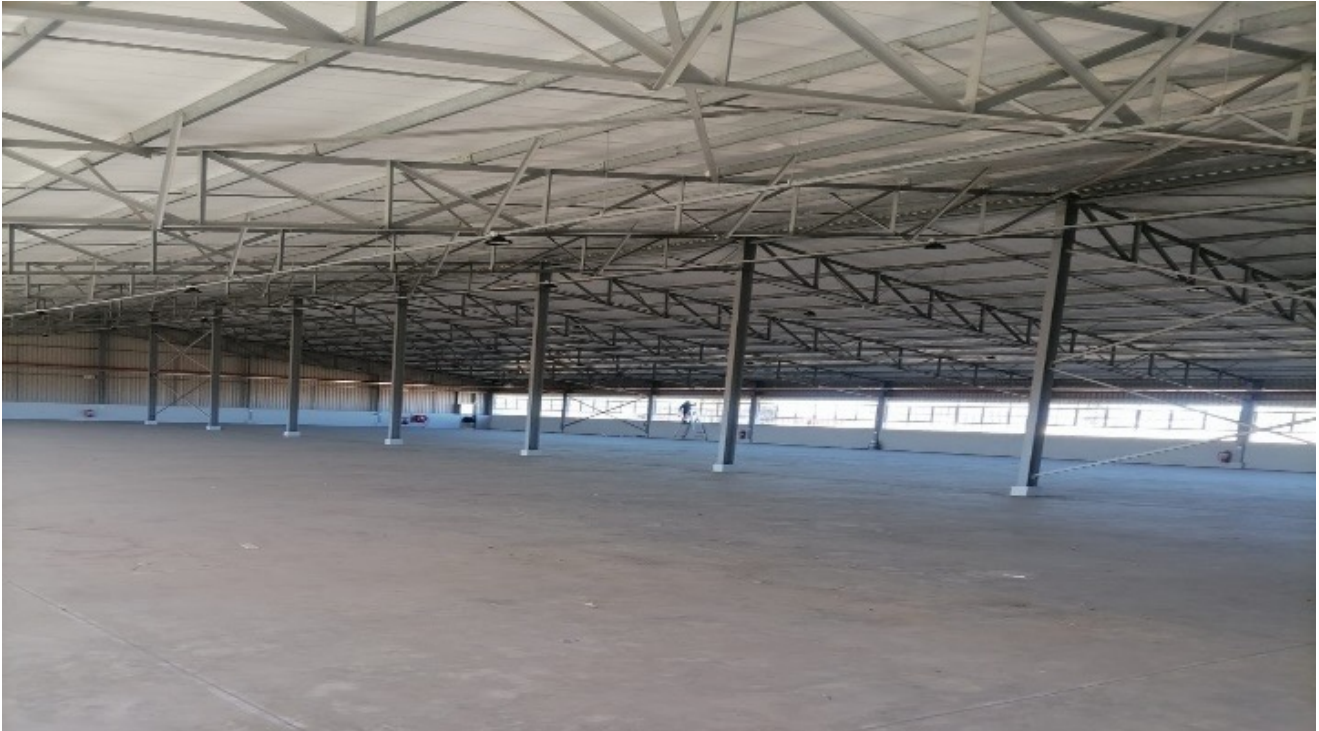
Rebuilt Factory at the Madadeni Industrial Estate
