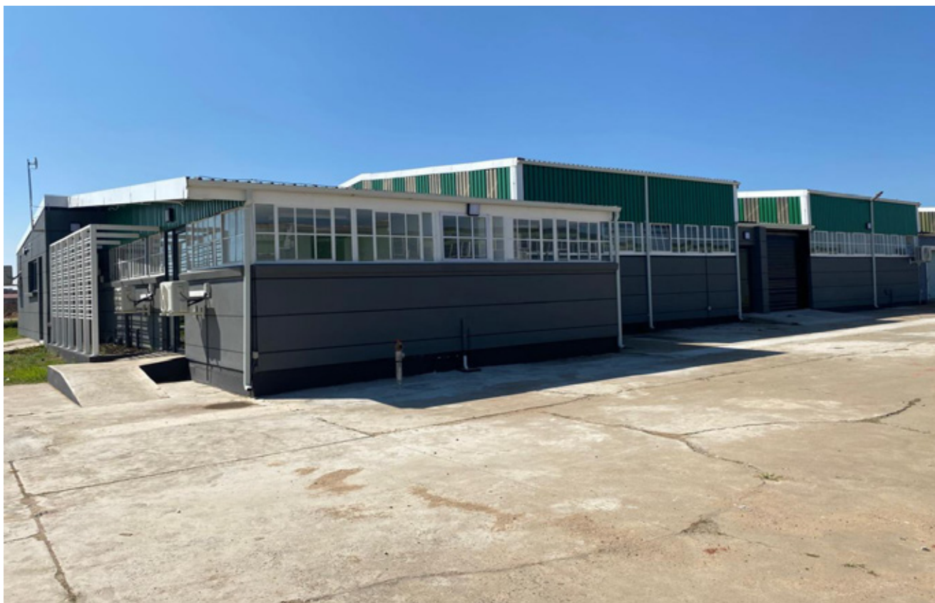
Newly established Vula Detergents Share Manufacturing Facility in Madadeni, Amajuba District Municipality
