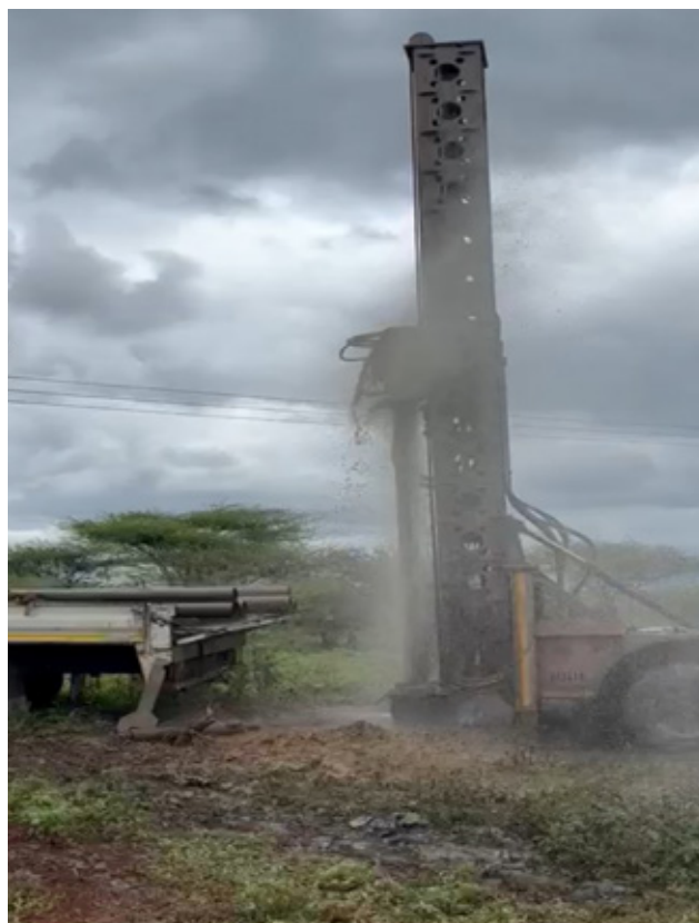
Borehole installation at the Ndumo Retail Centre site
