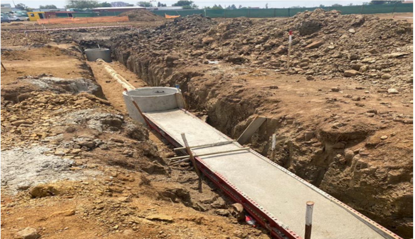
Start of Construction - Madadeni Clothing and Textile Hub, July 2023
