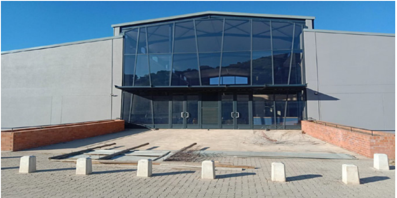
Tugela Ferry Shopping Centre: Entrance to Vendor Stall Area
