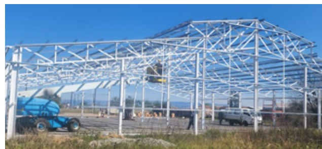
Ukwakhiwa kabusha eLot 50 eseMadadeni Industrial Estate
