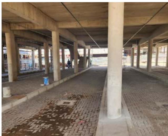
Newly constructed bus-bay at Tugela Ferry Taxi Rank
