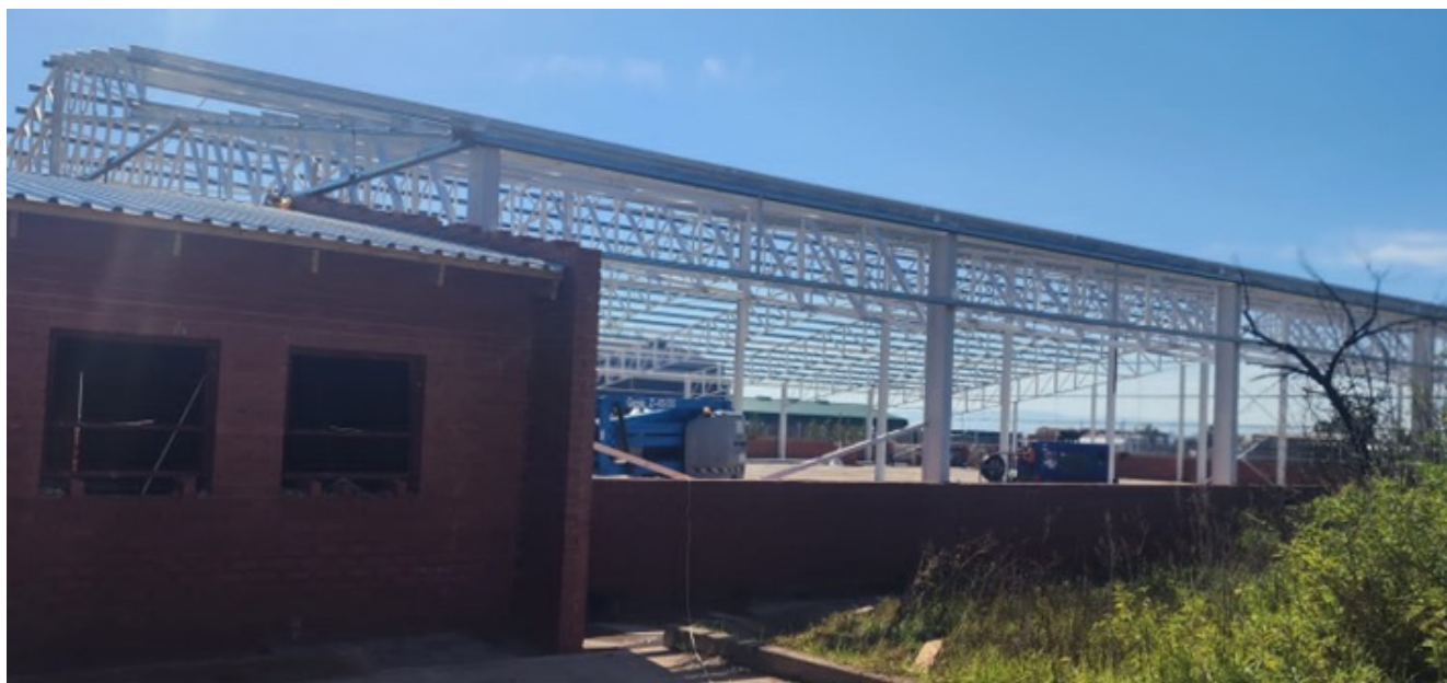
Rebuild at Lot 50 at Madadeni Industrial Estate
