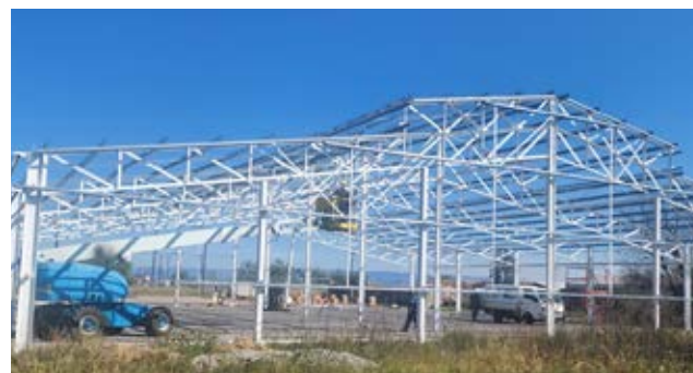
Rebuild at Lot 50 at Madadeni Industrial Estate
